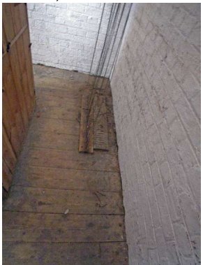
Above, is the second floor where the bell cables pass up from below.
