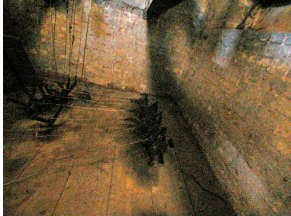
Above, is the third floor (very dark!) where the cables pass up from the space beneath and link to the bell cables.
